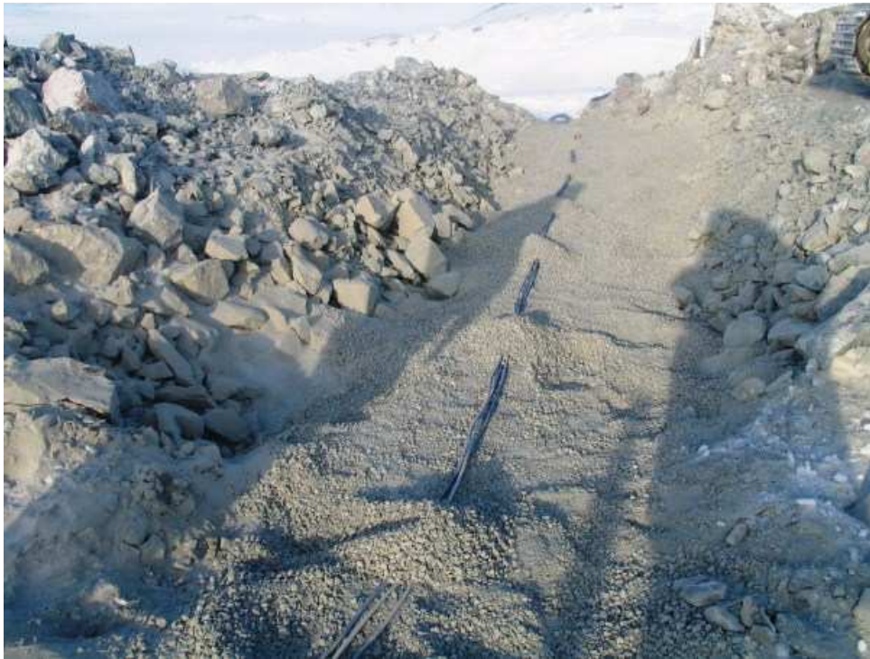
Photo 4: Bedding cables at Sta 1+75. Trench was cut in ramp
