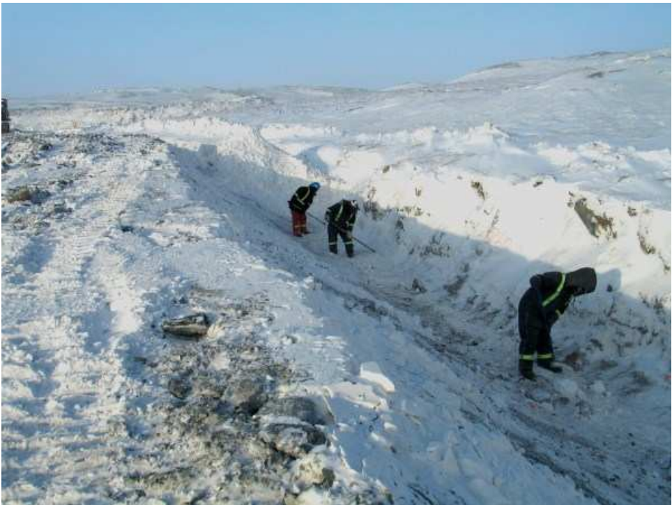
Photo 9: Cleaning bottom of key trench Sta 2+50 to 3+00
