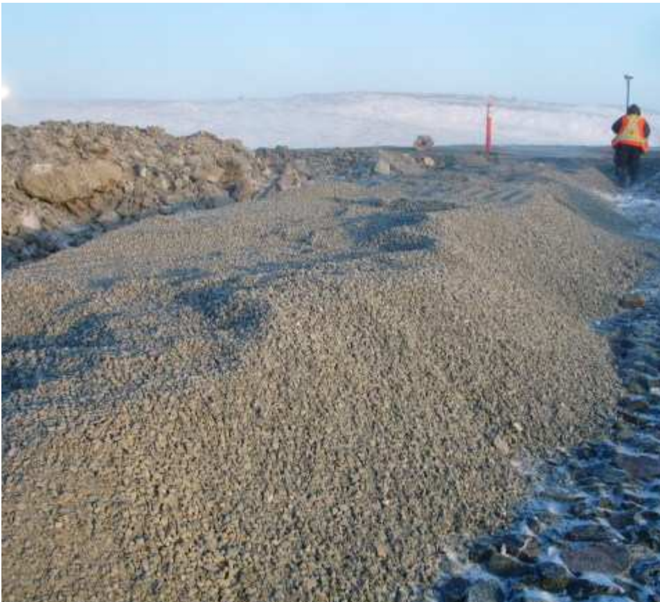
Photo 7: Final cover over cables at Sta 1+35
