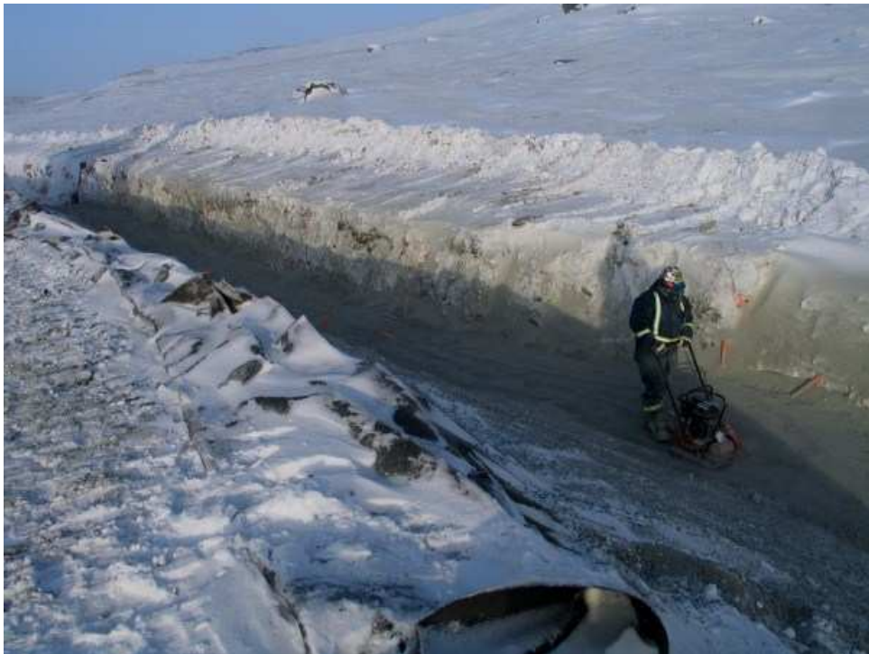
Photo 8: Packing bentonite between Sta 3+00 to Sta 3+35
