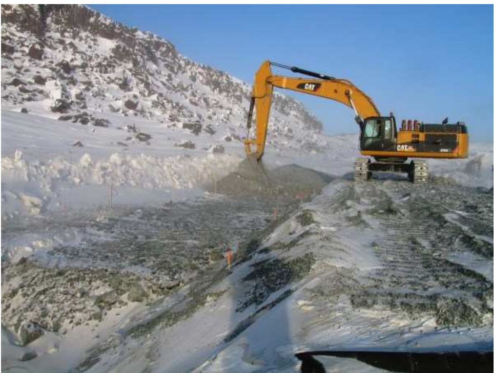
Photo 11: Placing second lift of ROQ ~ Sta 4+60
